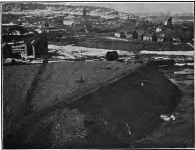
FIGURE 7 CLIFFS SHAFT MINE—CRUSHED ORE PILE, SHOWING METHOD OF FANNING OUT FROM TRESTLE
